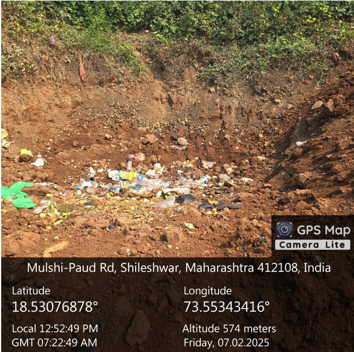
Kaccha compost pit -Permanent Pit not provided
